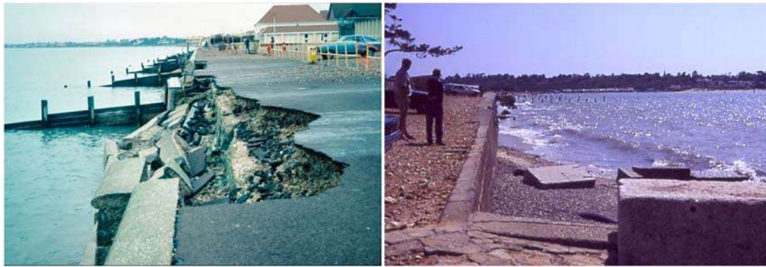
Fig. 3. Examples of structural failures and narrowed beaches in the 1980s on south coast of England.
